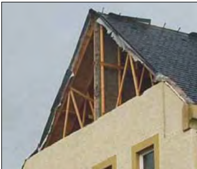
Fig 3.9: Gable wall failure
