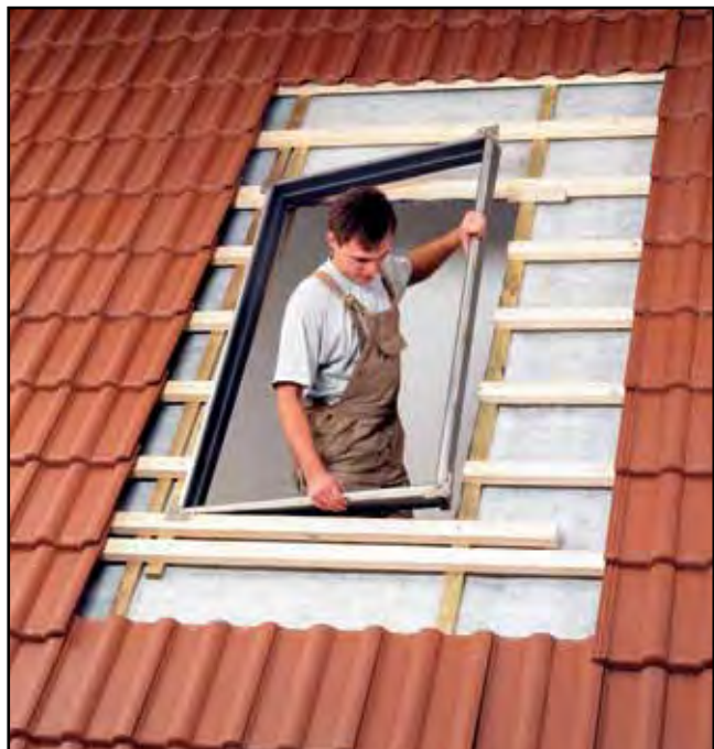
Fig 5.9: Inserting the support frame
