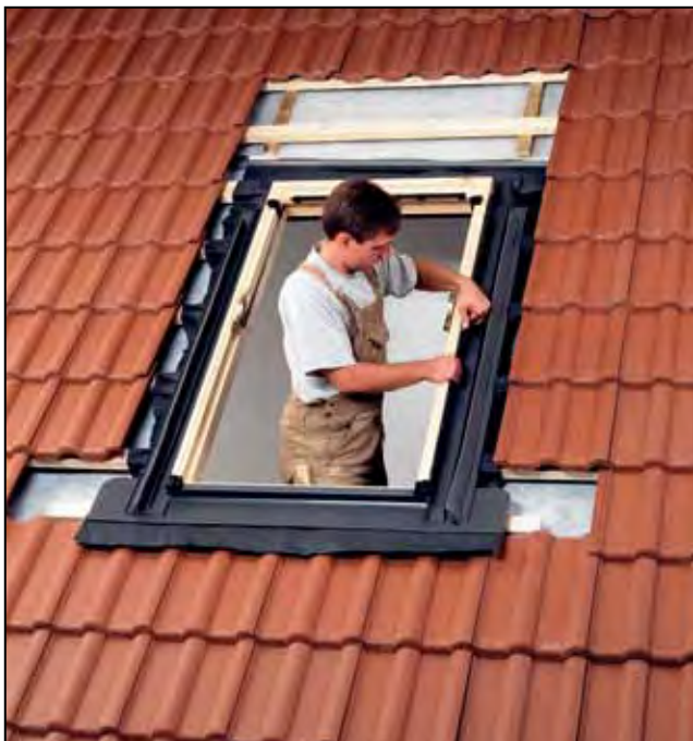
Fig 5.11: Installation of weatherproofing arrangement
