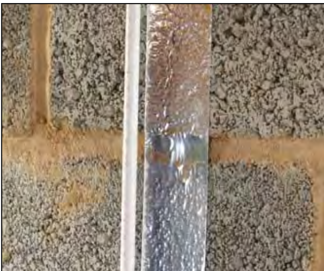
Fig 11.2: Positions for metallic tape by plastic pipes
