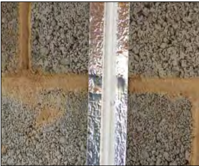
Fig 11.1: Positions for metallic tape by plastic pipes
