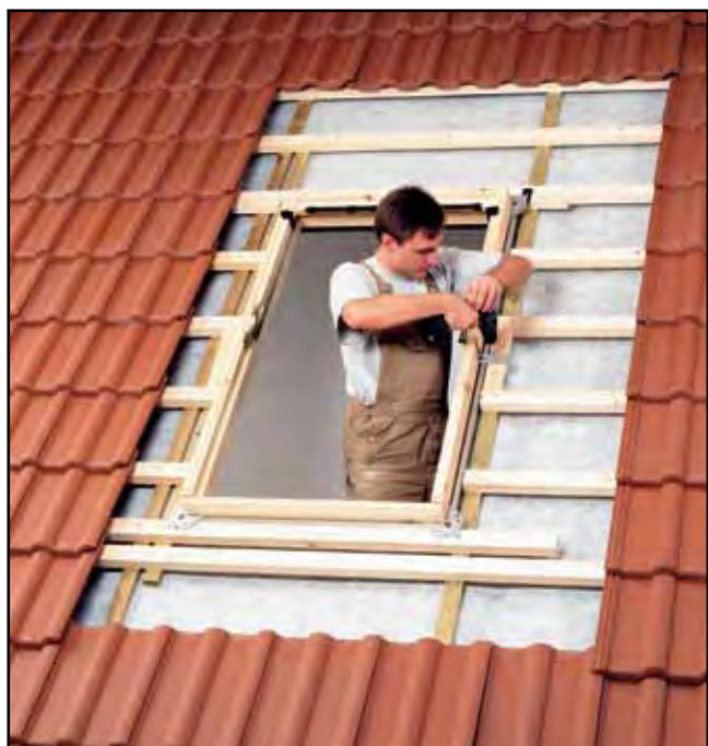
Fig 5.10: Securing the frame
