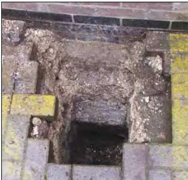
Fig 1 3.5: Trial hole for foundation inspection
